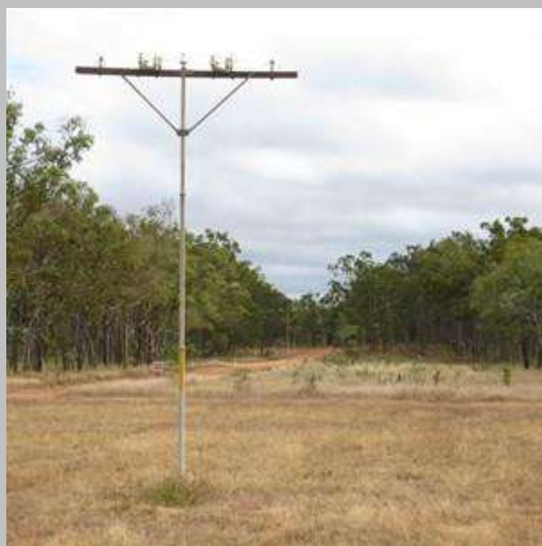
Original steel pole and insulators near the Moreton camping ground.
