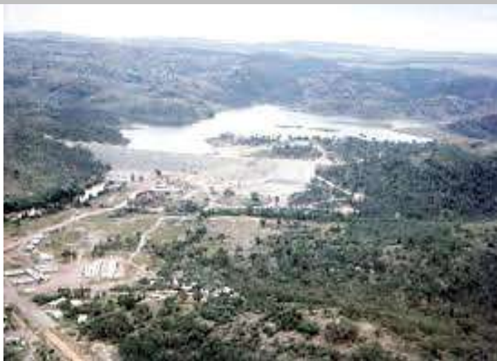
The Citra construction camp in the foreground of the near-completed dam.
