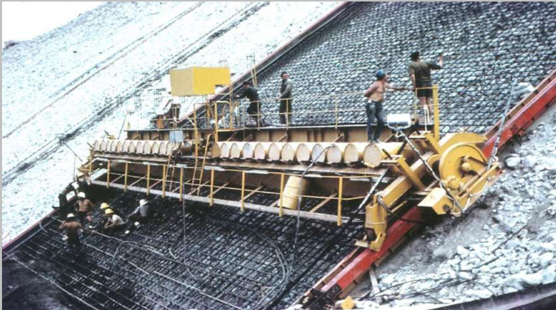
Facing the rock-fill dam with concrete, September 1968.
