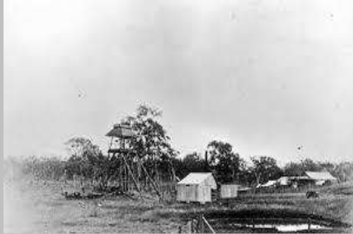
The Company's Reef mine was where the Calliope Sportsground is today
